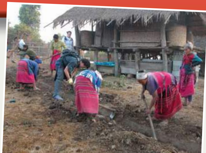
Laying the water supply pipeline.
