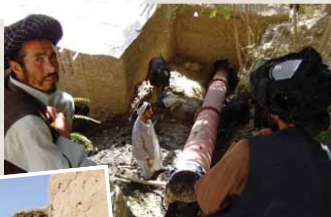
Installation of pipes to control water flow.
