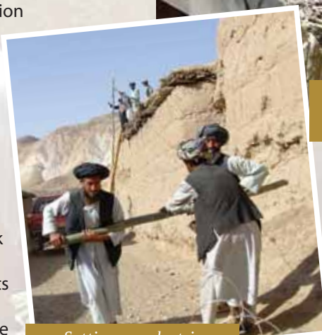
Setting up electric distribution lines.
