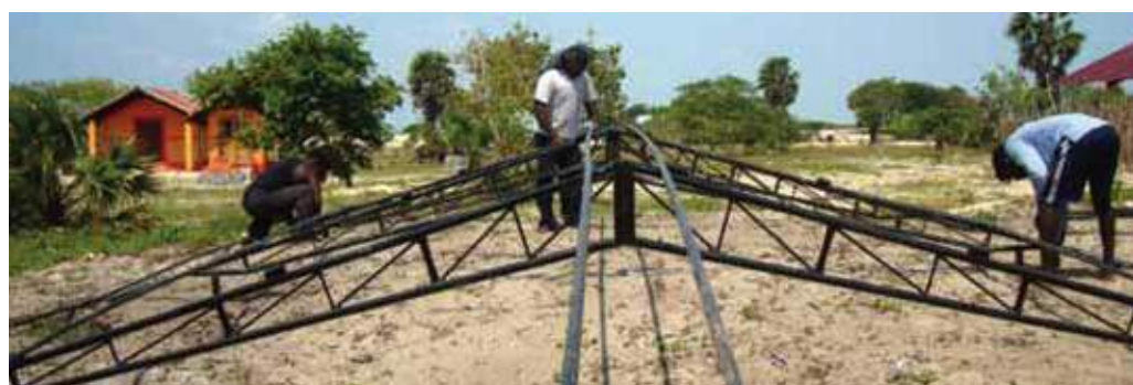
Roof beams for the new community hall
