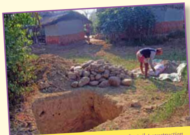
Prem Bahadur Katuwal preparing cement for toilet construction
