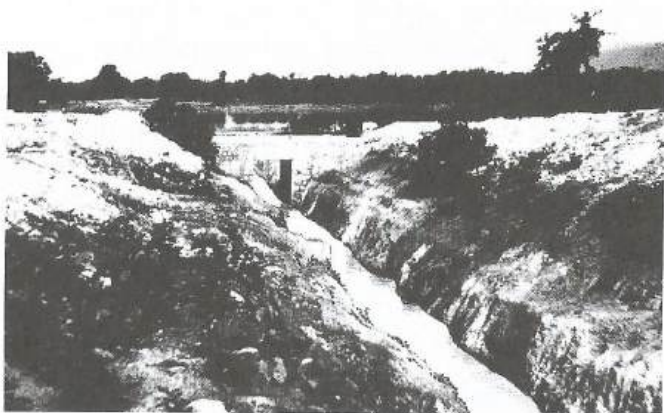
The scale of this Diptipur "Food for Work" irrigation canal can be judged by the white cow to the right of the bridge
