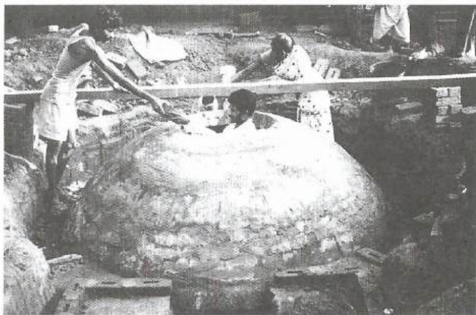
Putting the finishing touches to a village bio-gas plant near Diptipur
